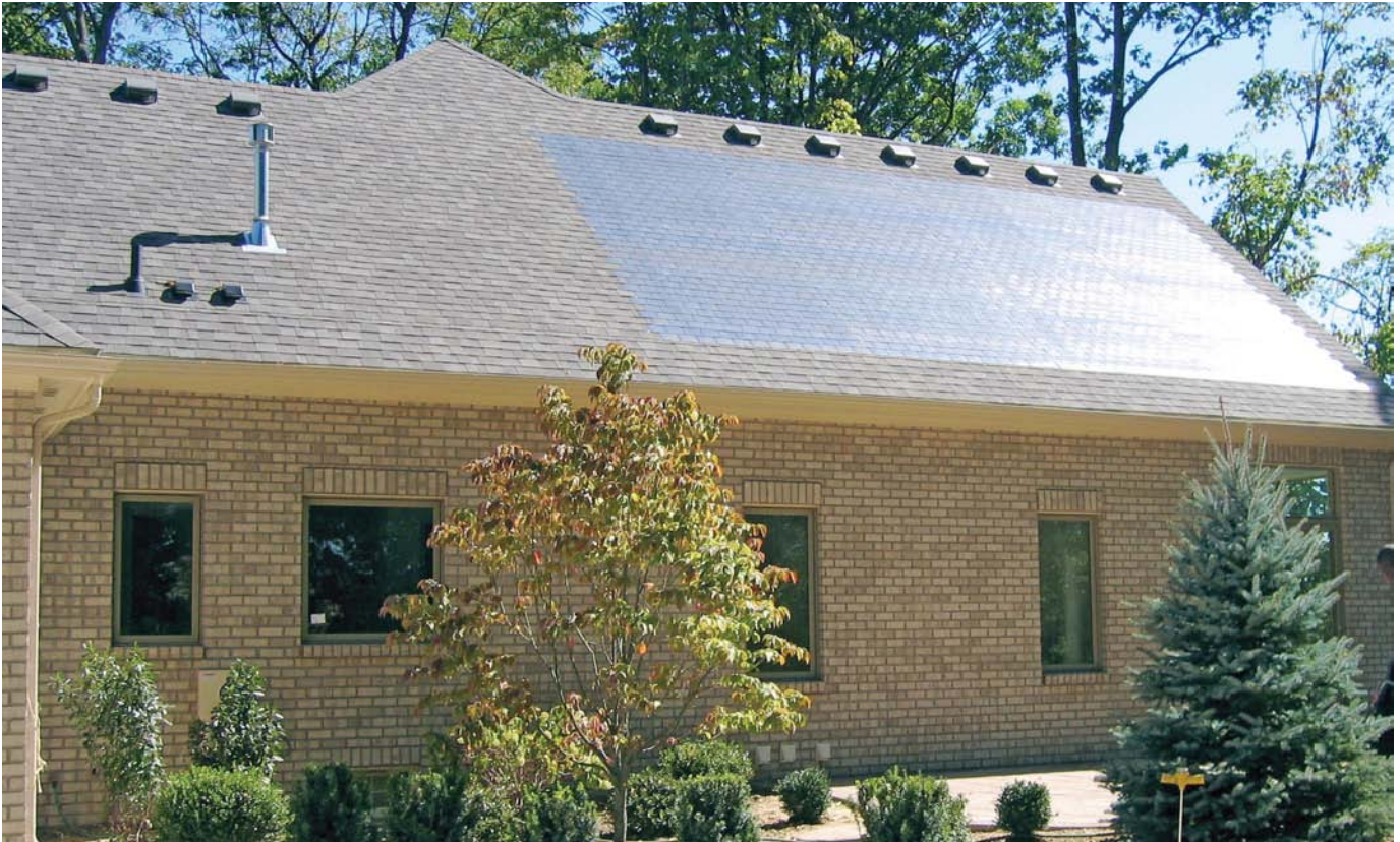
PV shingles seamlessly blend into this home's rooftop, merging form with function.
