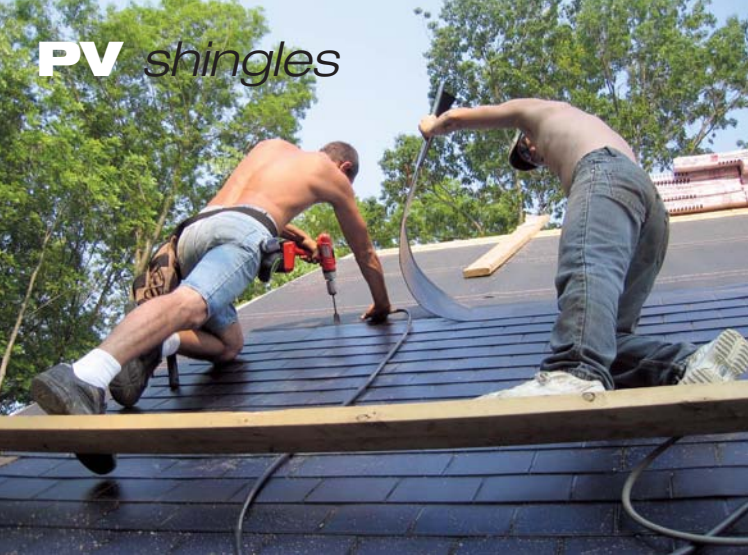
Drilling the wiring holes before nailing the PV shingles.
