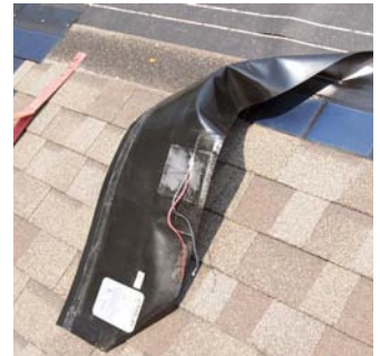
Below: Wiring leads on the back of a PV shingle.
