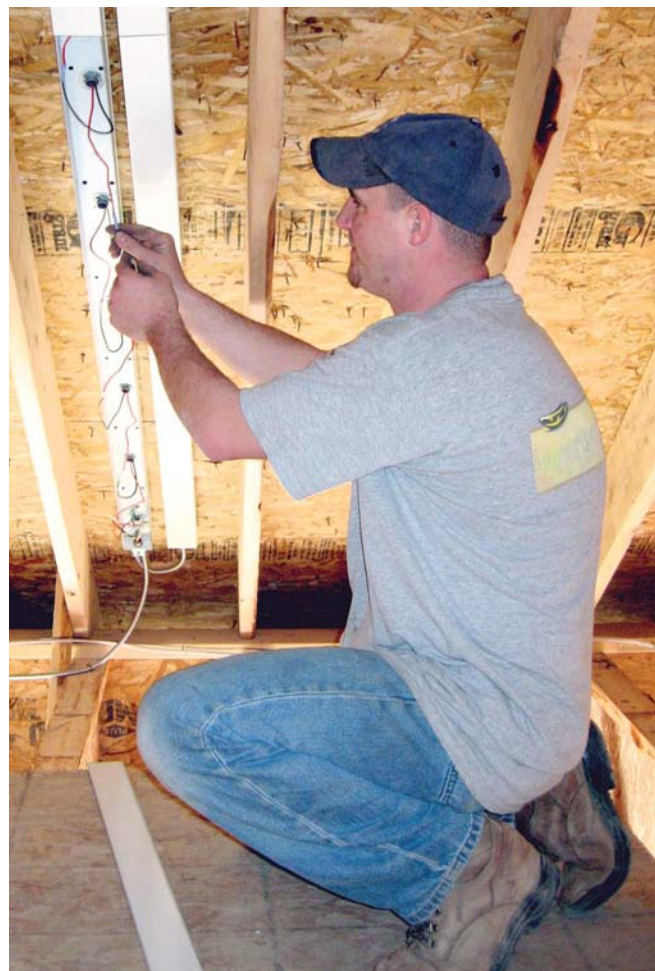
Making series connections in the raceway.
